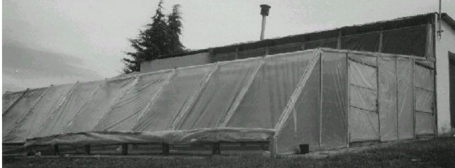
Figure 1: Solar dryer located in Northern Portugal - Mirandela
